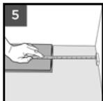
At the end of the first row, put a spacer to the wall and measure the length of the last panel to fit.
